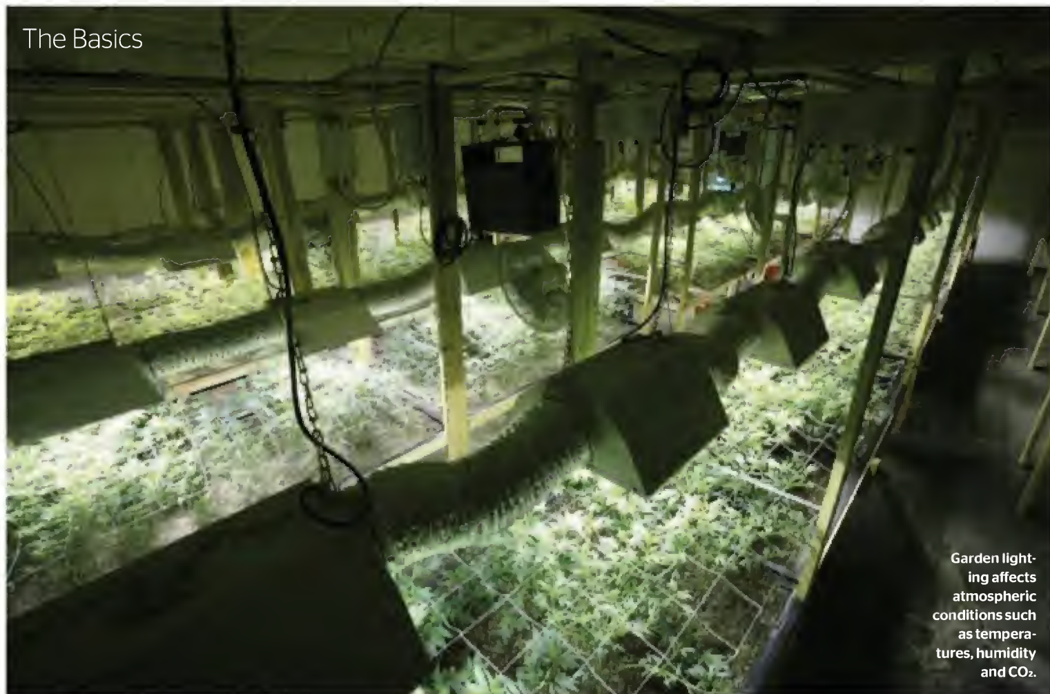
Lamp hoods with glass lenses and side flanges for air-cooling help control environment conditions.
